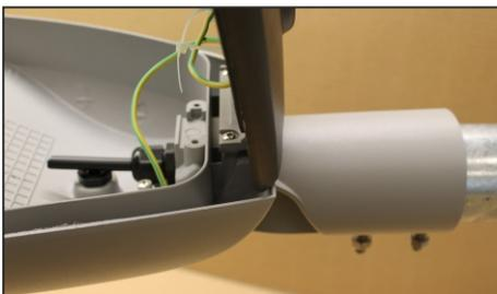
11. Make sure that the luminaire is correctly horizontally installed. Tighten two Allen screws with tightening torque of 8 Nm and secure with nuts
