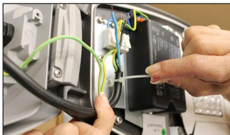
14. Connect the wires to the terminal block:
