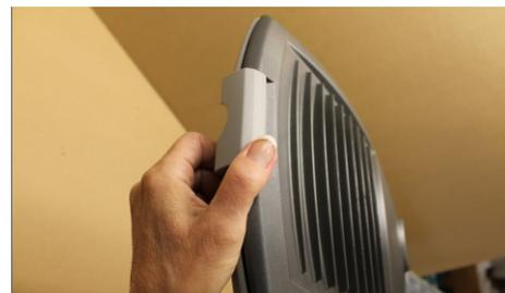
18. Orientation of the luminaire for the post instalation.
