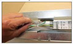
7. Electrical connection of the terminal block
