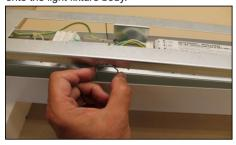
2. Slide the cover of the housing by pushing it.
