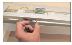
6. Connect the cable to the terminal block.
