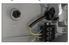
11. Strip the end of the cable (7 cm) and the ends of the wires (1 cm)
